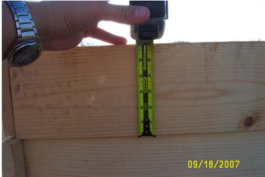
Figure 3: Lumber support frame (1x8 cut down to exactly 6" wide)
