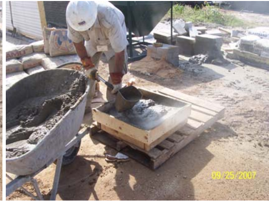
Figures 11 and 12: Application of sprayed mortar into wooden forms
