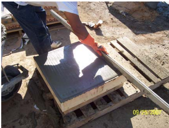
Figures 13 and 14: Smoothing of mortar in wooden form
