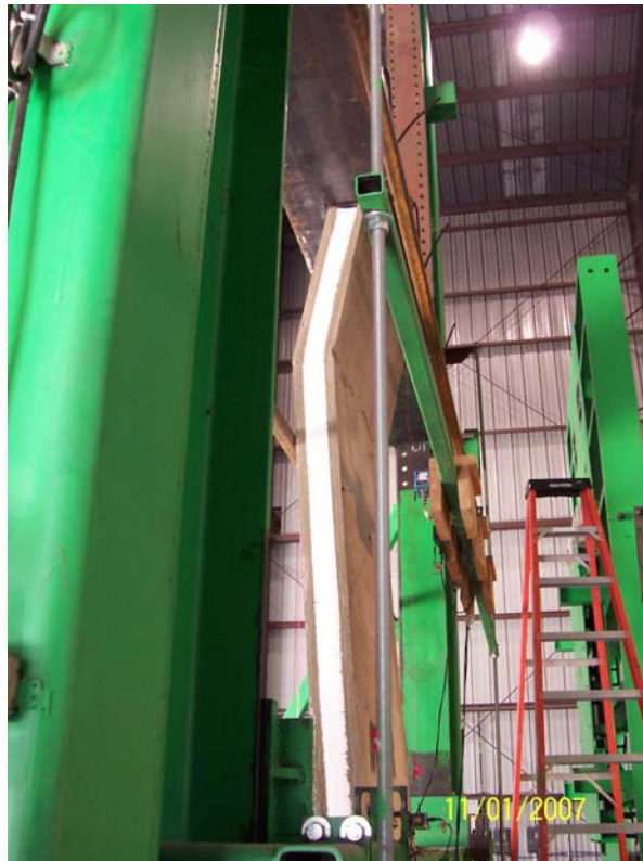
Figure 4A: 4X8A1 Failure mode
