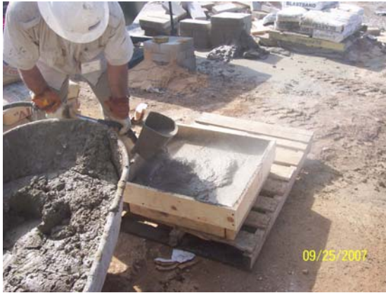
Figures 11 and 12: Application of sprayed mortar into wooden forms
