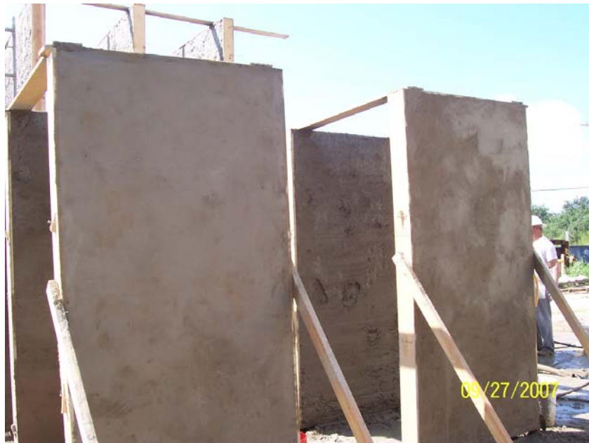
Figure 7: Finished 4' x 8' PSM80 wall panels
