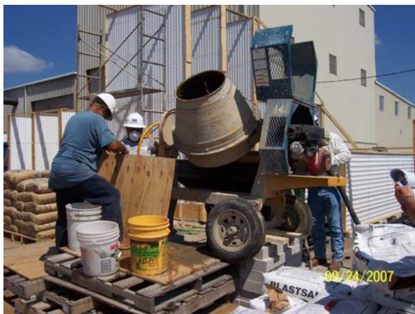
Figures 4 and 5: Mortar mixing and spraying application on wall assemblies, respectively
