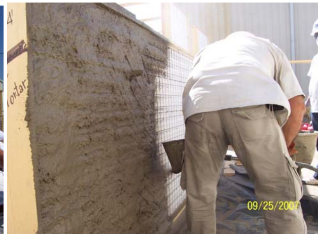
Figures 4 and 5: Mortar mixing and spraying application on wall assemblies, respectively
