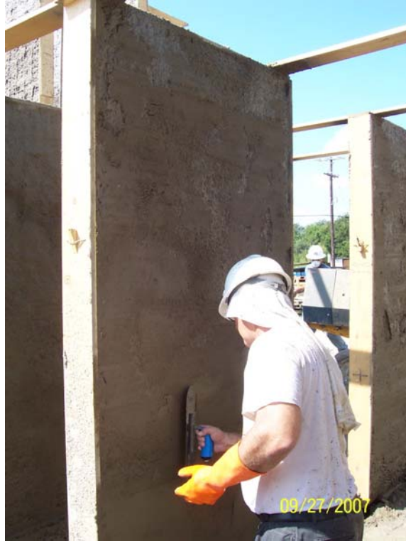
Figure 6: Smoothing out mortar after spraying
