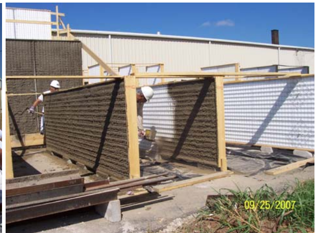
Figures 4 and 5: Mortar mixing and spraying application on 4' x 14' wall assemblies, respectively
