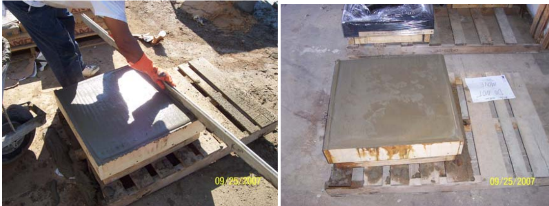
Figures 15 and 16: Smoothing of mortar in wooden form
