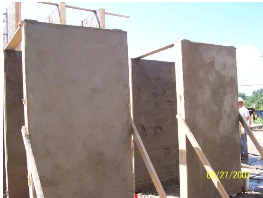
Figure 7: Finished 4' x 8' PSM80 wall panels
