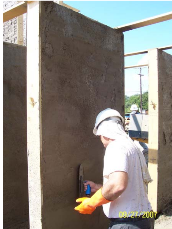
Figure 6: Smoothing out mortar after spraying
