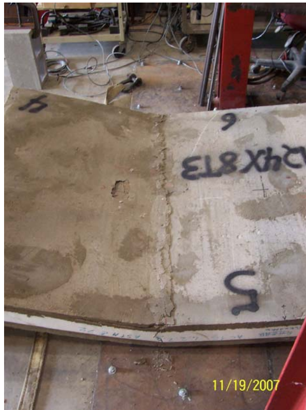
Figure 4A: 4X8T3 Failure mode (close-up)
