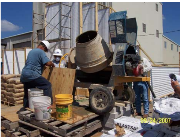
Figures 4 and 5: Mortar mixing and spraying application on 4' x 14' wall assemblies, respectively
