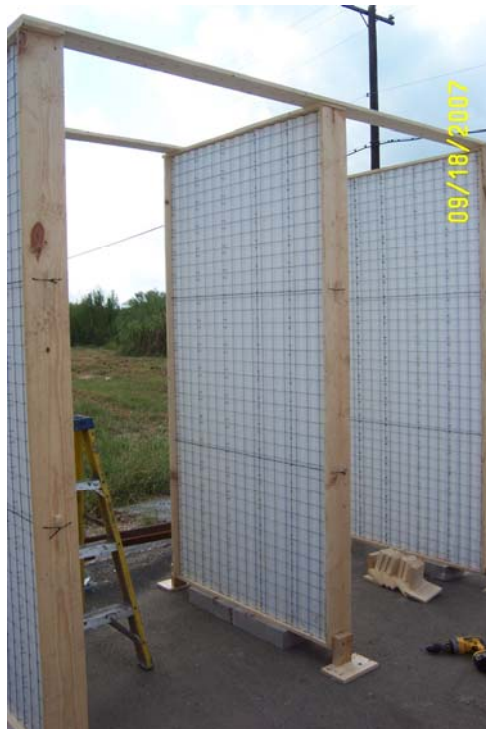
Figure 2: Finished wood frames with 4' x 8' panels ready for spray mortar application
