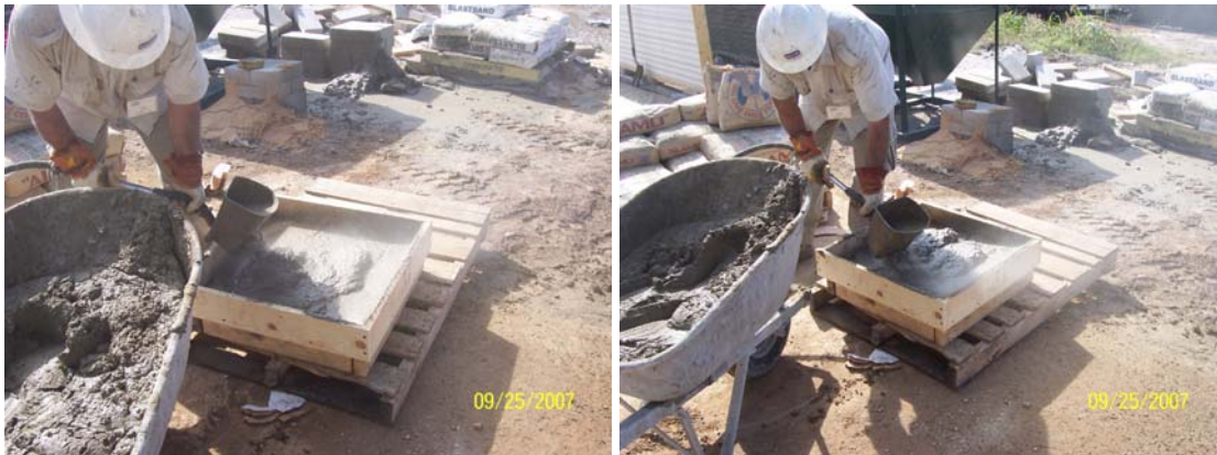
Figures 14 and 15: Application of sprayed mortar into wooden forms
