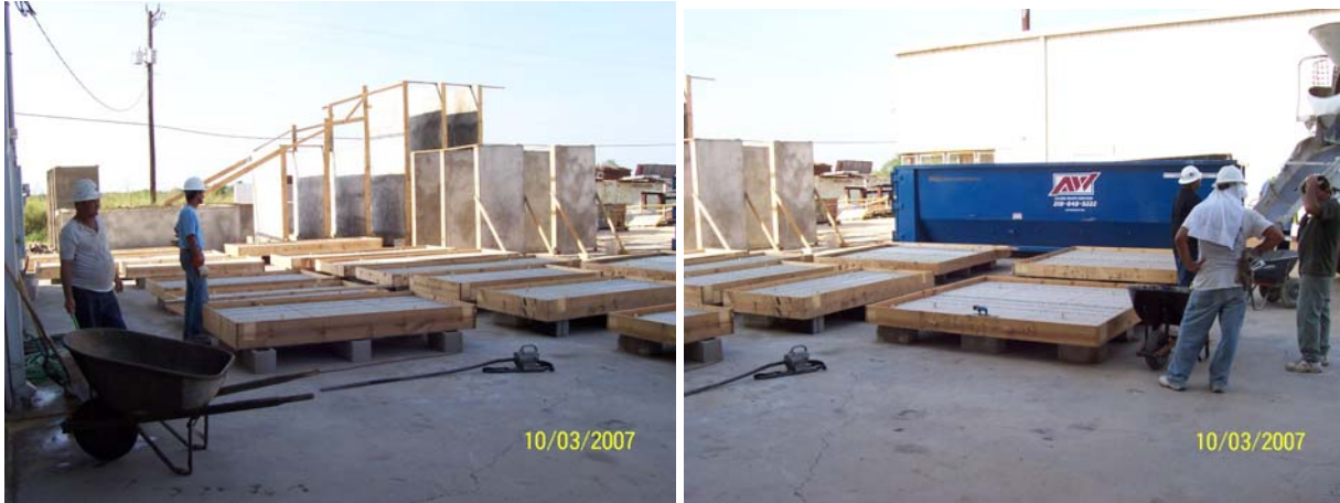
Figures 5 and 6: Floor/roof panels prepared for concrete pouring
