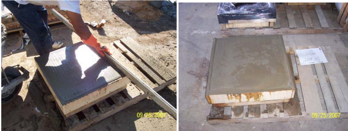
Figures 16 and 17: Smoothing of mortar in wooden form
