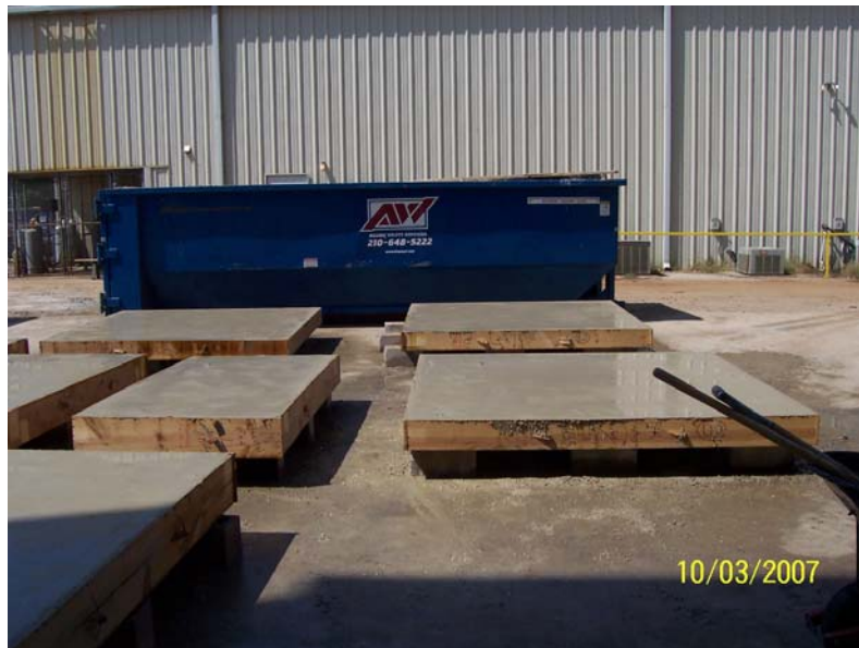
Figure 7: Finished floor/roof panels with concrete wetted down
