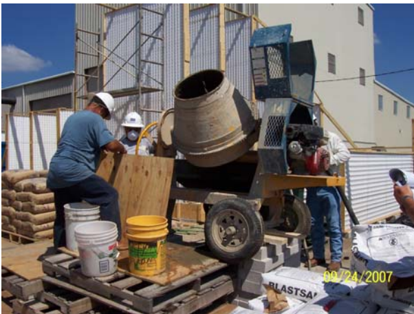
Figures 3 and 4: Mortar mixing and spraying application on 4' x 12' assemblies, respectively
