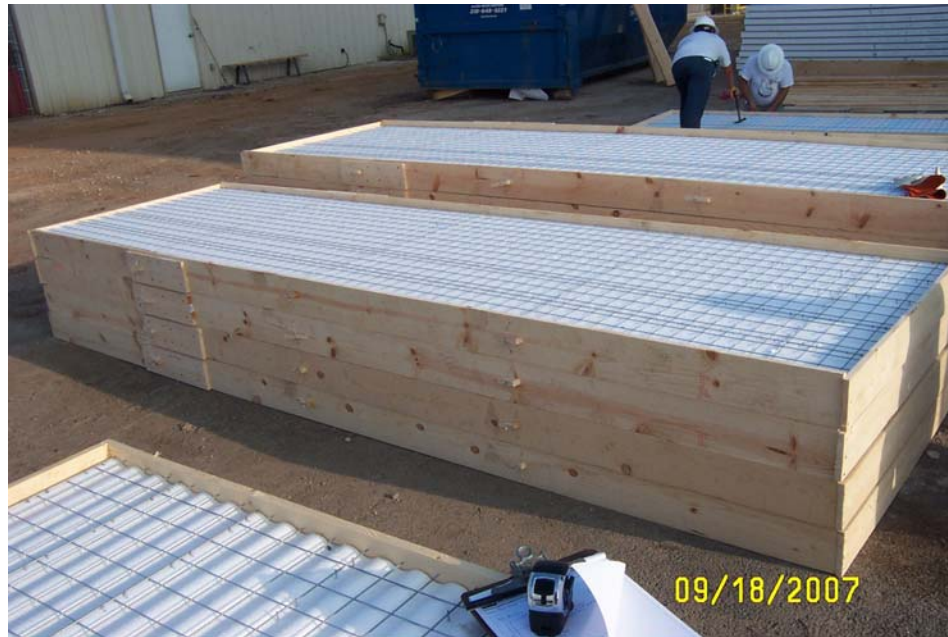
Figure 2: Finished wood frames with 4' x 12' panels ready for spray mortar application
