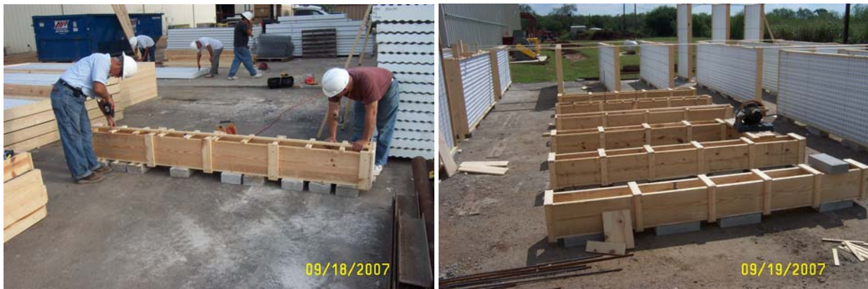
Figures 2 and 3: Wooden molds prior to rebar installation
