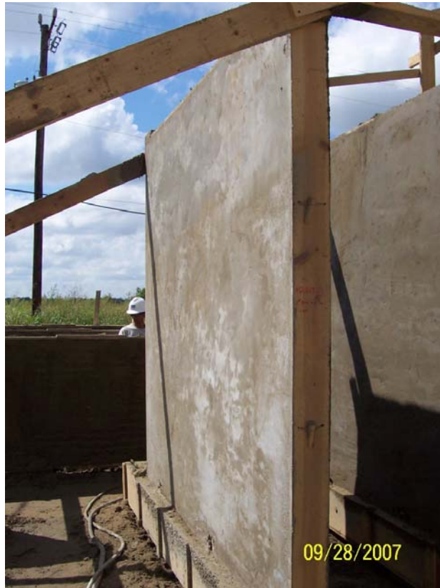
Figure 22: Finished 8' x 8' shear panel
