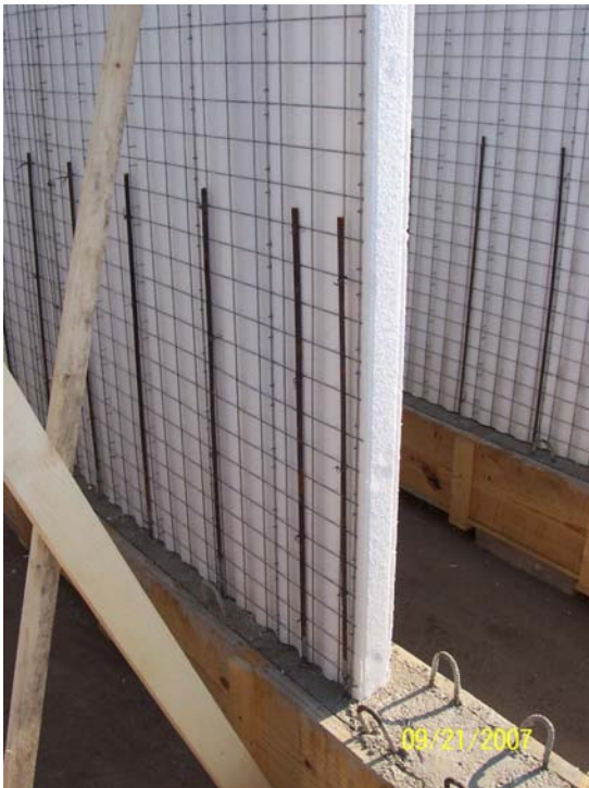
Figures 16 and 17: Finished rebar connections into panel wire mesh prior to perimeter frame installation
