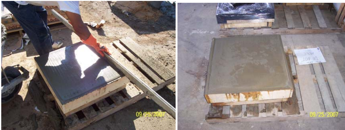
Figures 33 and 34: Smoothing of mortar in wooden form
