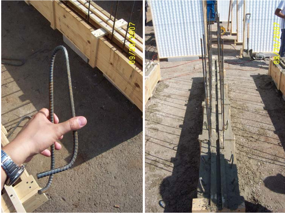
Figures 10 and 11: #5 rebar hook (approx 3" wide x 13" long) and finished footer
