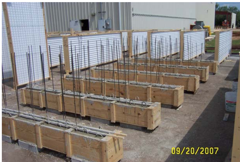
Figure 12: Finished shear wall footers
