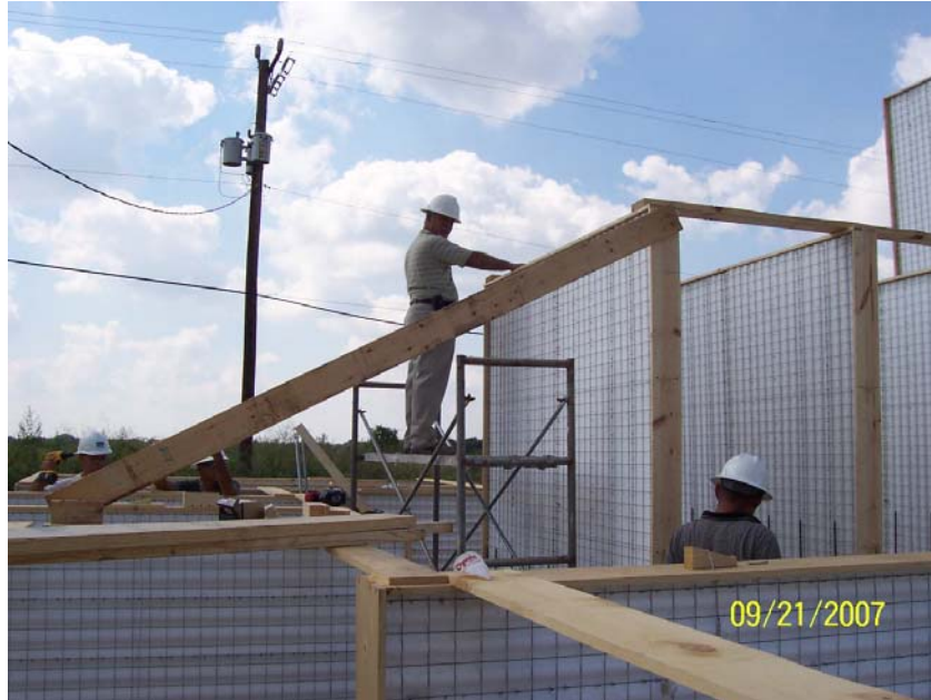
Figure 18: Finished 8x8 shear wall with perimeter frame and stabilizers
