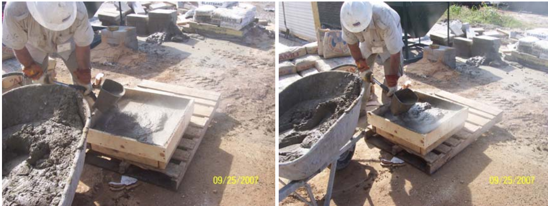
Figures 31 and 32: Application of sprayed mortar into wooden forms
