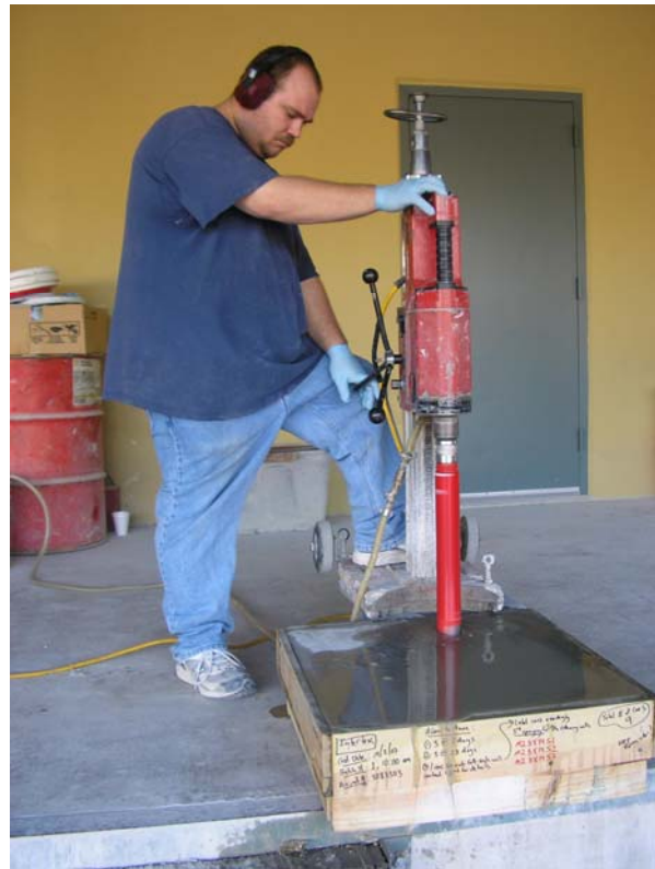
Figure 37: Drilling of mortar cores
