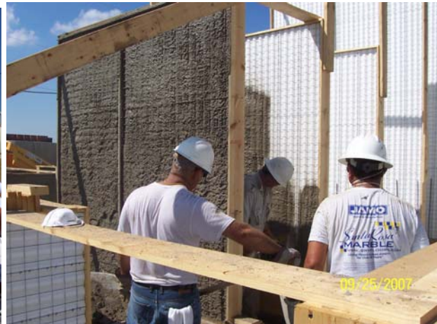
Figures 19 and 20: Mortar mixing and spraying application on wall assemblies, respectively
