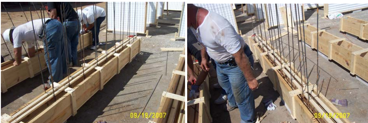
Figures 8 and 9: Finished installation of rebar
