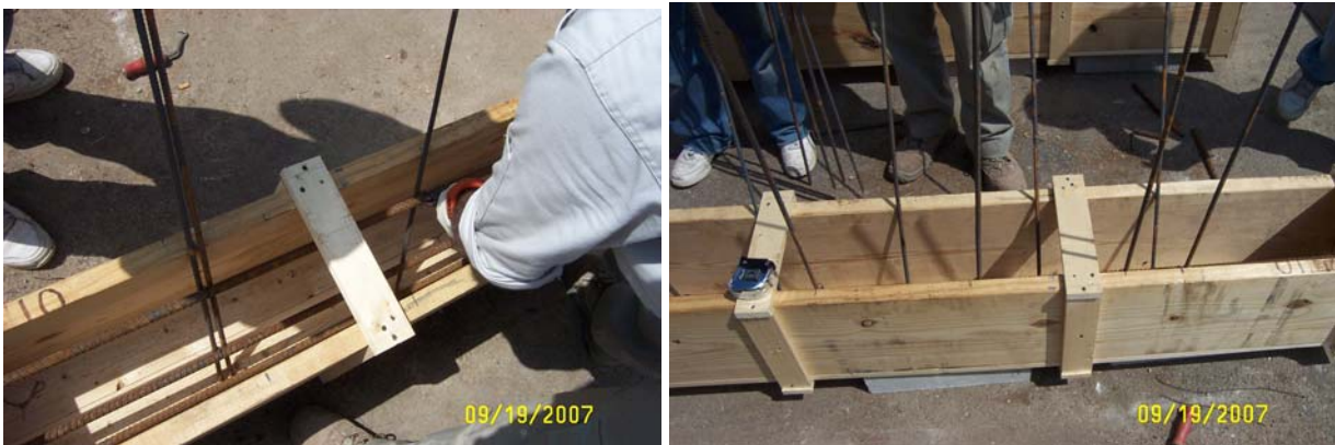
Figures 6 and 7: Installation of vertical #3 rebars into footer
