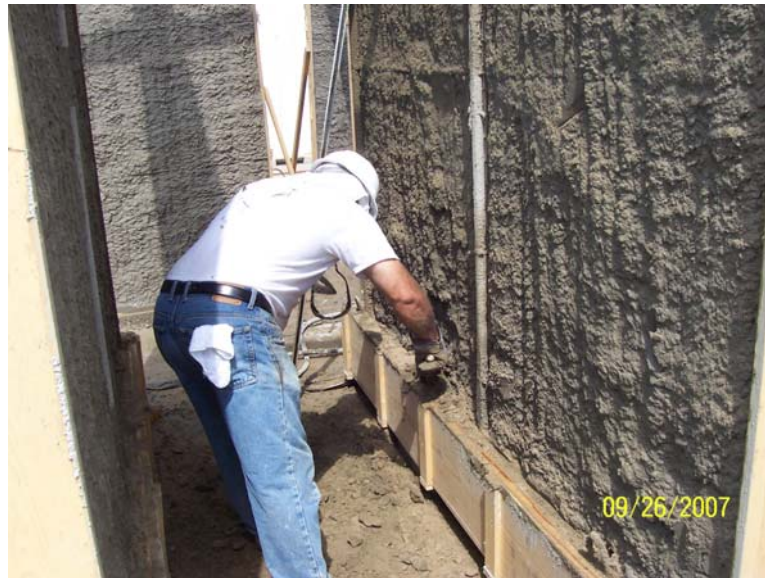
Figure 21: Smoothing out mortar after spraying
