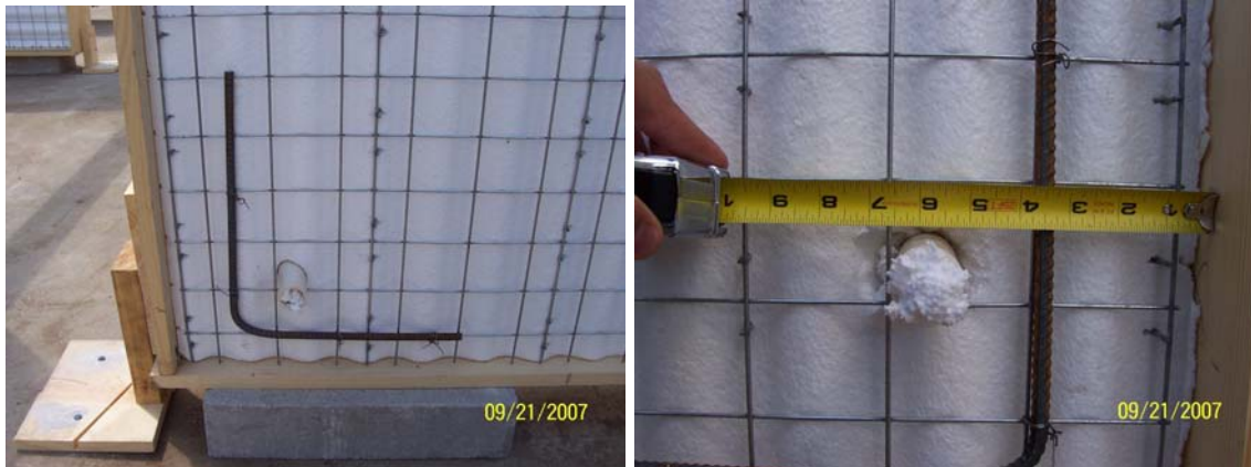
Figures 6 and 7: Installation of #3 rebar at hinge location (both sides)
