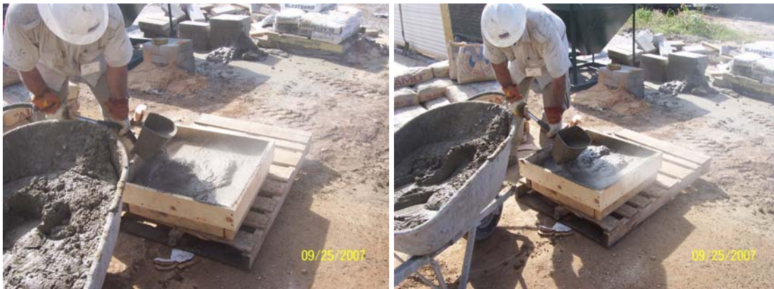
Figures 23 and 24: Application of sprayed mortar into wooden forms
