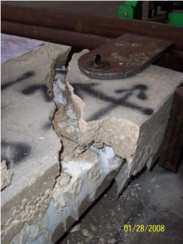
Figure 6A: Failure mode (close-up)
