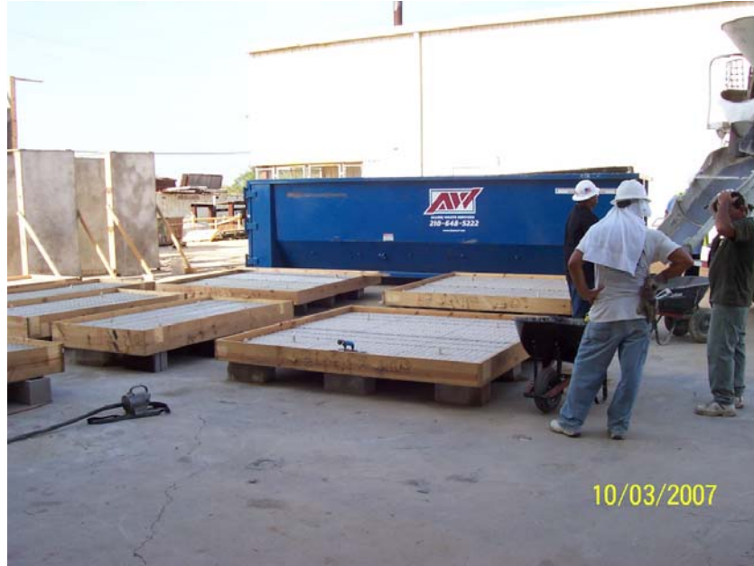
Figure 13: Diaphragm shear samples before concrete pour
