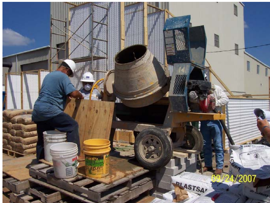
Figure 9: Mortar mixing
