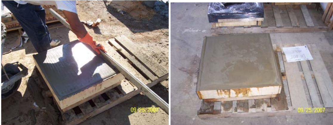
Figures 25 and 26: Smoothing of mortar in wooden form
