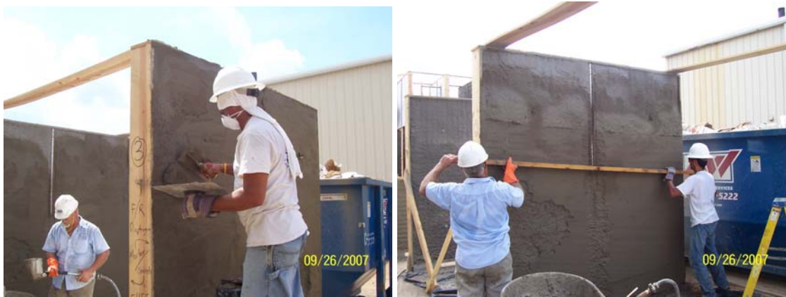
Figures 11 and 12: Smoothing of mortar
