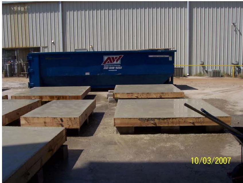
Figure 14: Diaphragm samples after concrete pour
