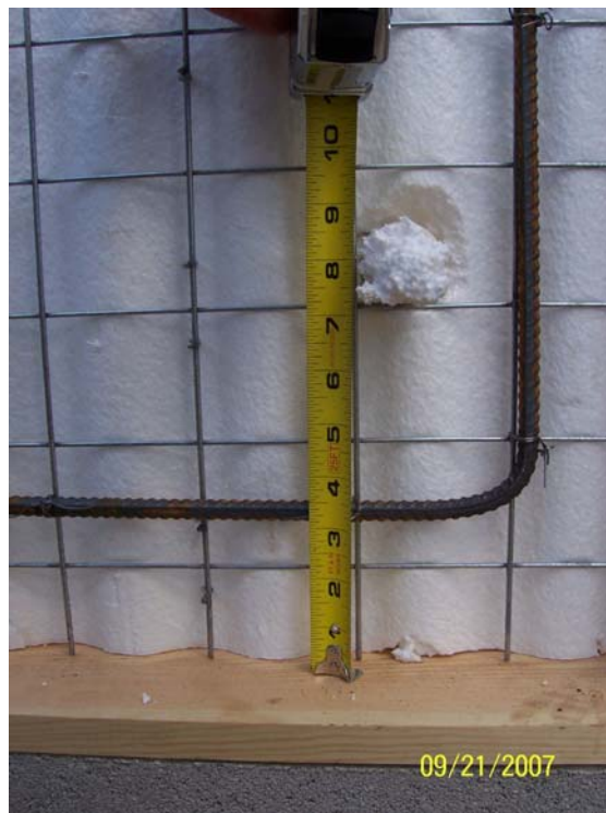
Figure 8: Rebar at hinge (concrete side)
