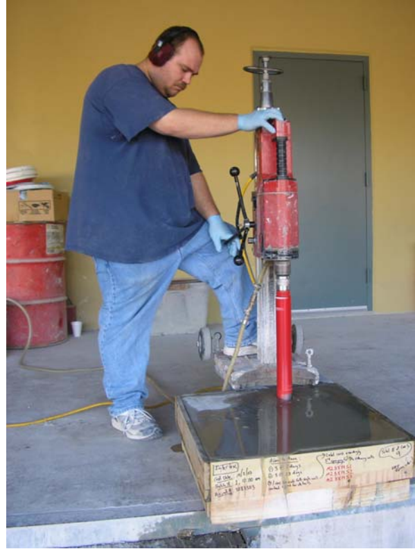
Figure 29: Drilling of mortar cores
