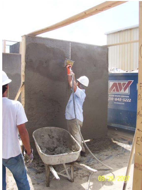
Figure 10: Spraying application of diaphragm samples
