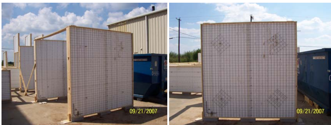
Figures 2 and 3: Finished framework and supports for diaphragm panels
