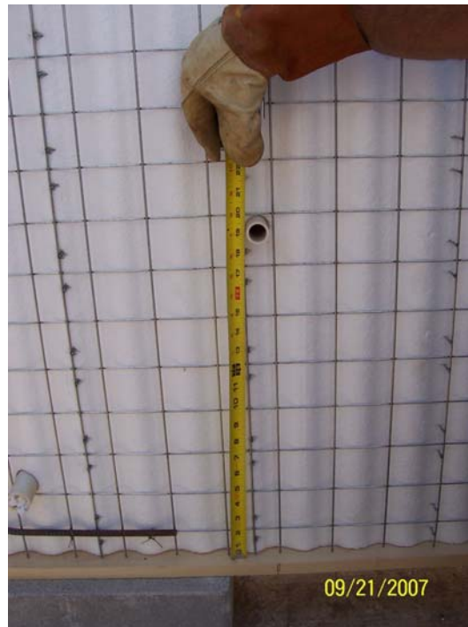
Figure 10: Location of lifting point from bottom
